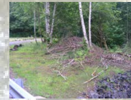
An example of stockpiling soil in situ from bridge replacement excavations because of the presence of an invasive weed in the area. The weed has since been removed but the soil will not be re-spread until the land managers are sure there is no chance of a reemergence.
